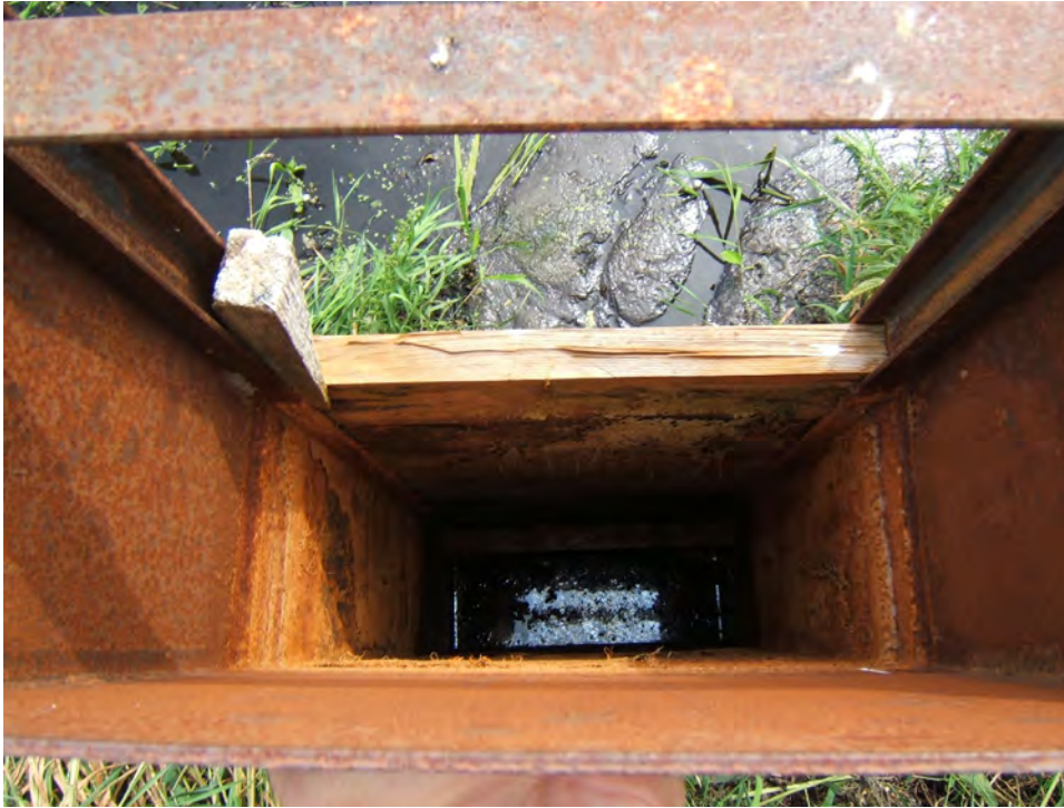
Figure 23. Main Line Tile Outlet Structure
