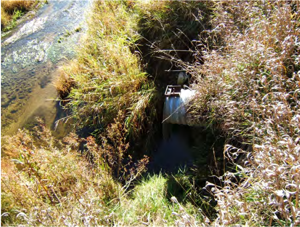
Figure 17. Culvert at Sparby Monitoring Site From Which Samples Are Collected
