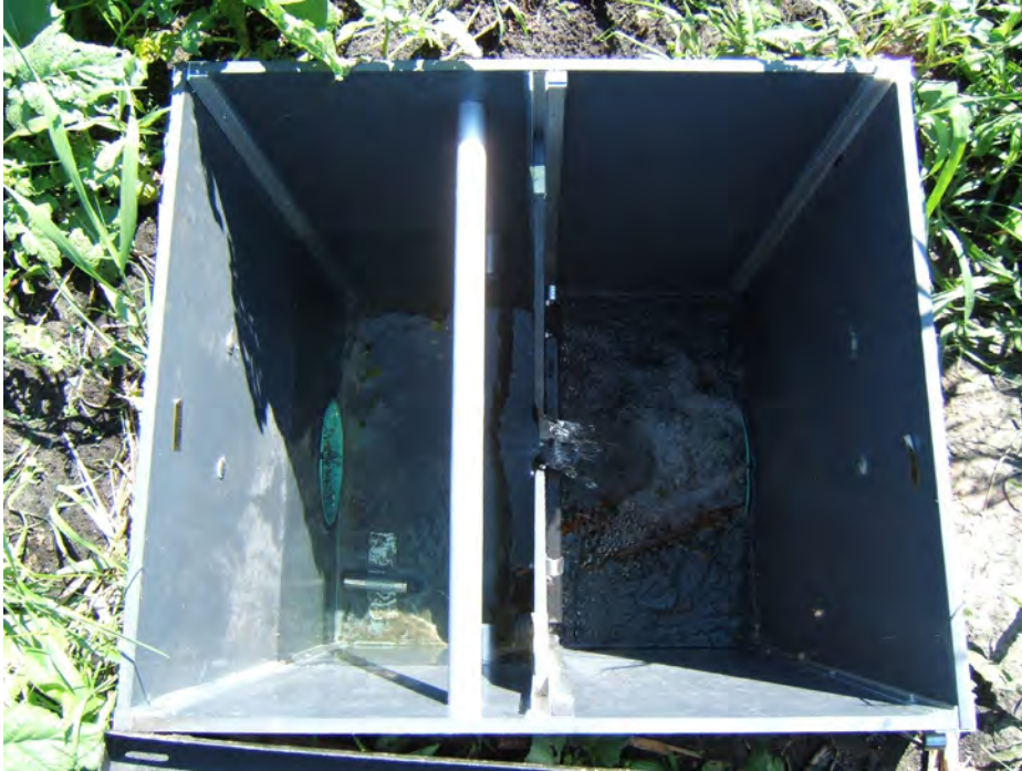
Figure 3. Bachand Tile Drainage Water Control Structure
