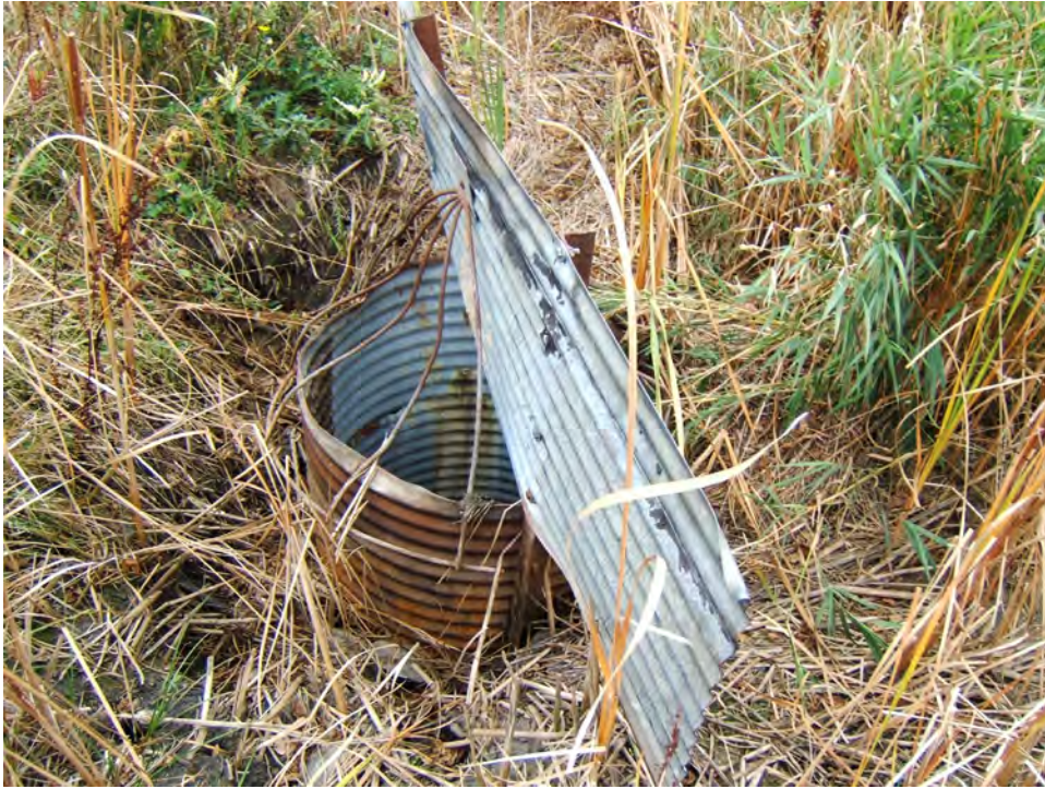
Figure 11. Drop Structure at the Upstream End of Yaggie 1 Culvert
