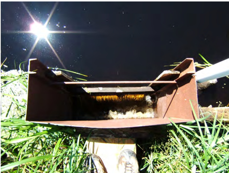
Figure 20. Surface Drained Wild Rice Paddy Outlet Structure
