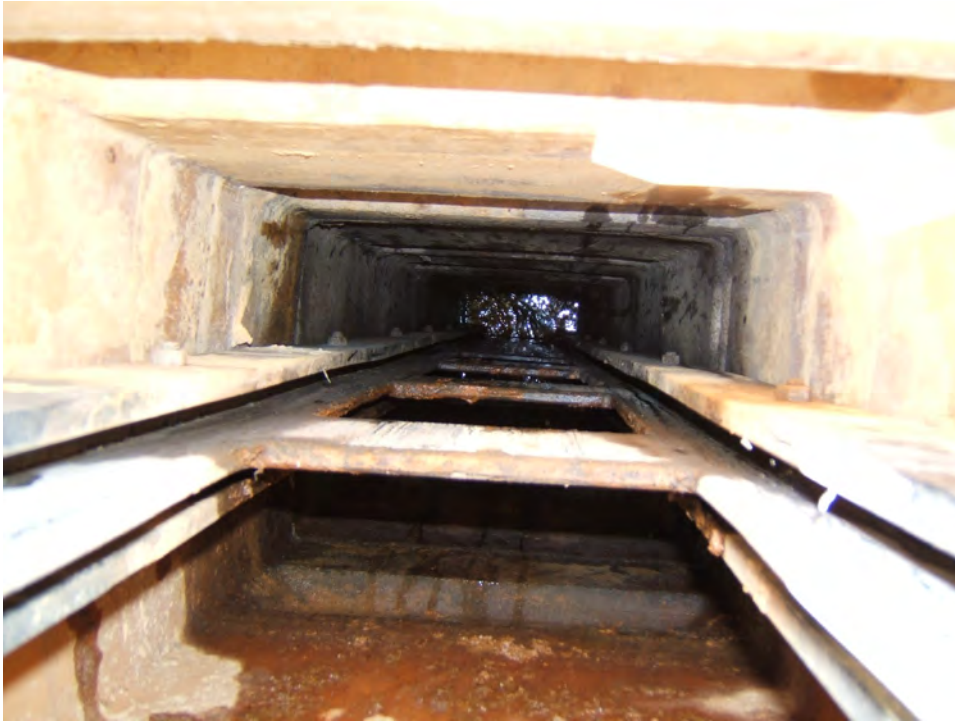
Figure 2. View down a Clearwater Rice Main Line Tile Water Control Structure
