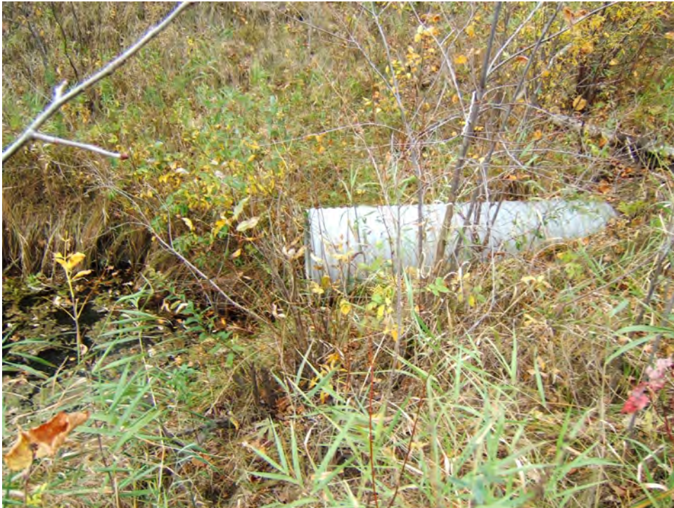
Figure 10. Downstream End of Yaggie 1 Culvert
